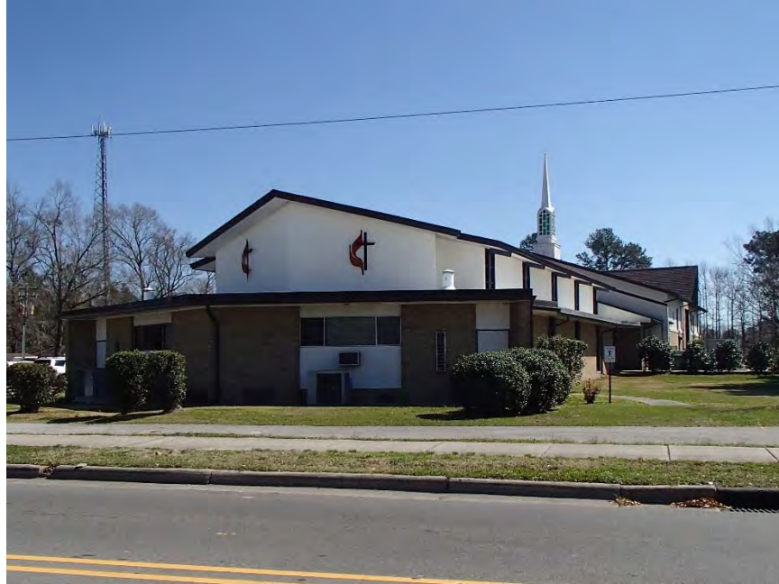
Figure 11: Northwoods UMC, northwest elevation
