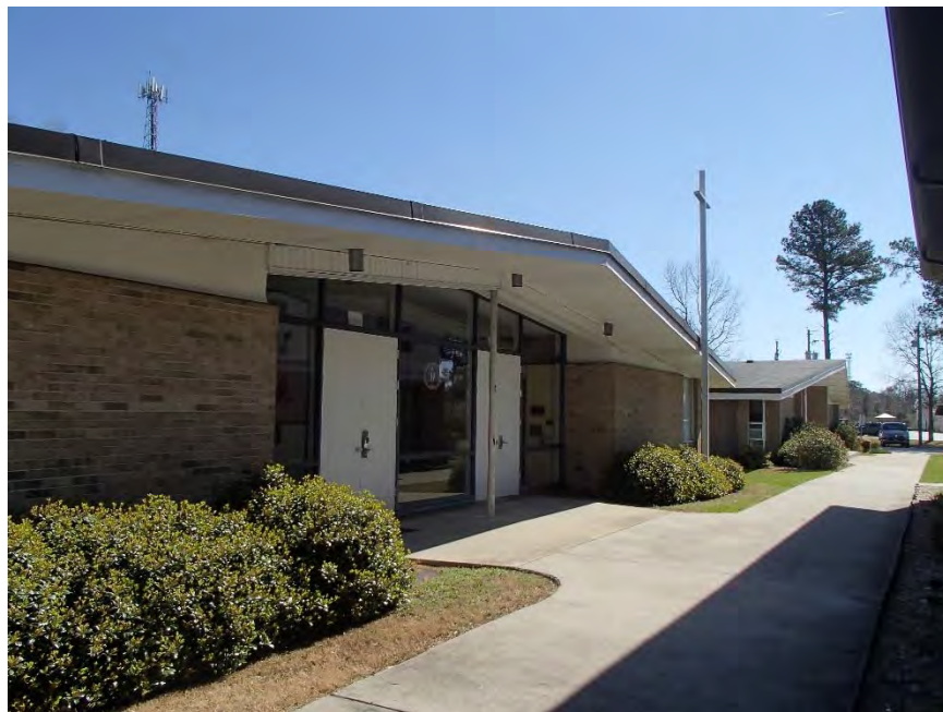
Figure 8: Northwoods UMC, Education Building, southwest elevation
