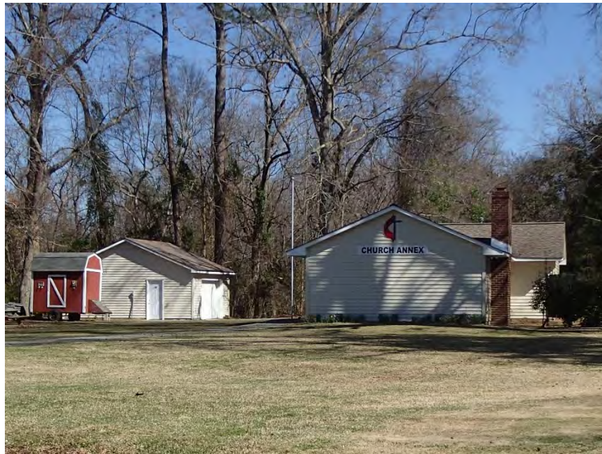
Figure 32: Northwoods UMC, Annex and Garage, facing northeast
