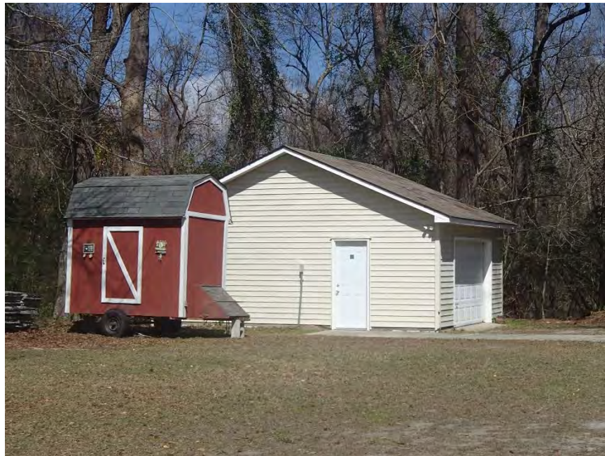
Figure 34: Northwoods UMC, Garage, southwest elevation
