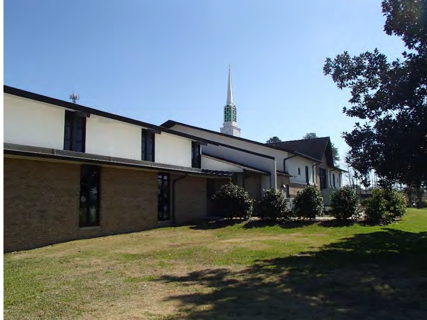
Figure 13: Northwoods UMC, southwest elevation, from Fellowship Hall toward 2008 sanctuary
