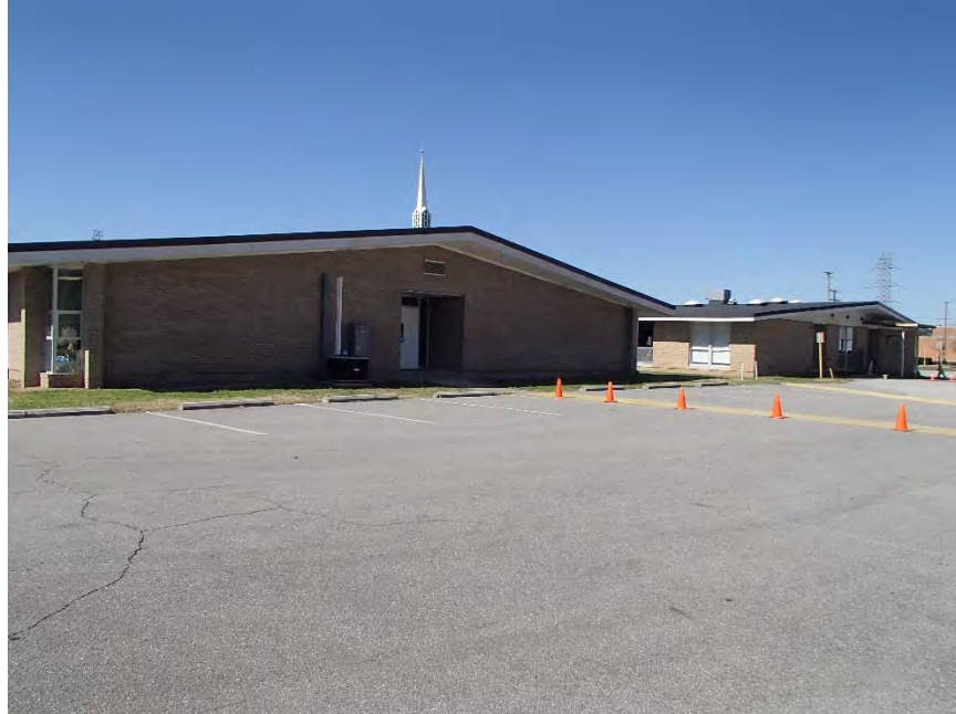
Figure 29: Northwoods UMC, Second Education Building, northeast elevation
