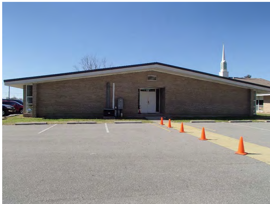
Figure 30: Northwoods UMC, Second Education Building, northeast elevation
