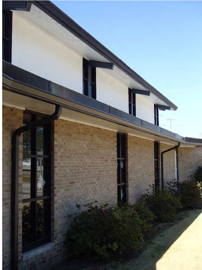
Figure 21: Northwoods UMC, Fellowship Hall exterior detail
