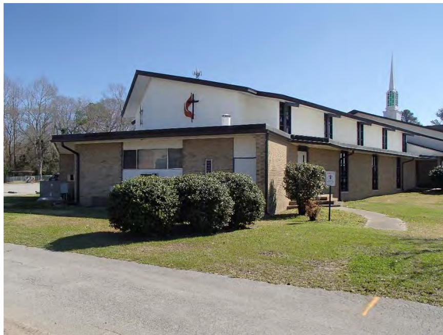
Figure 10: Northwoods UMC, Fellowship Hall, west corner
