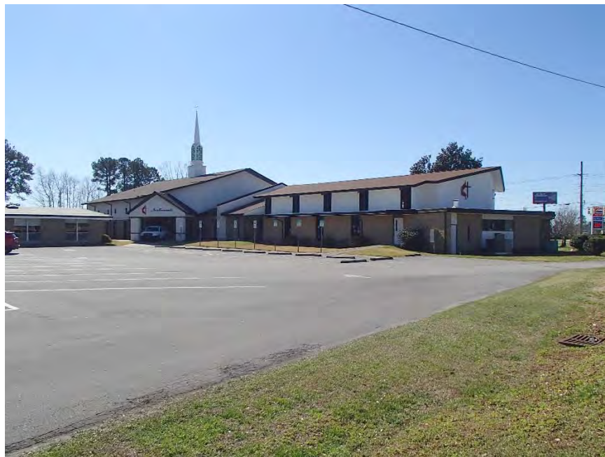
Figure 20: Northwoods UMC, north corner and northeast elevation
