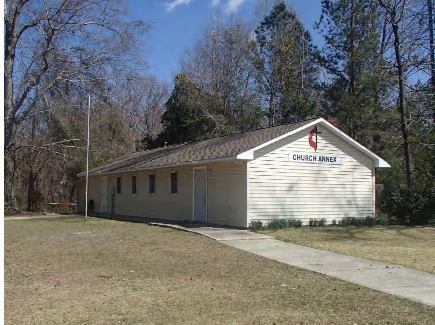
Figure 33: Northwoods UMC, Annex, west corner
