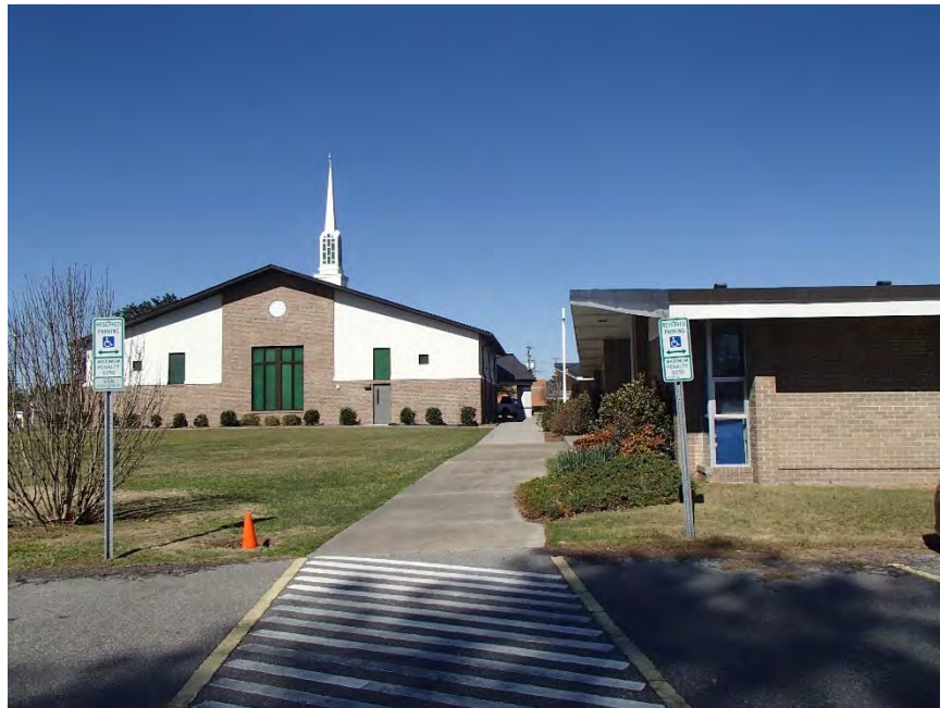
Figure 18: Northwoods UMC, southeast elevation with Education Building
