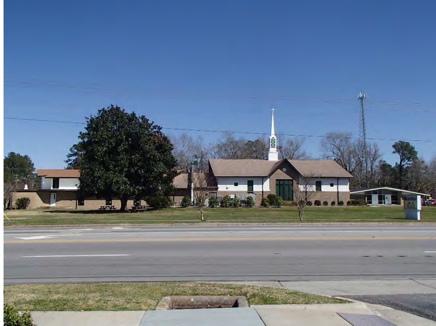
Figure 15: Northwoods UMC, southwest elevation
