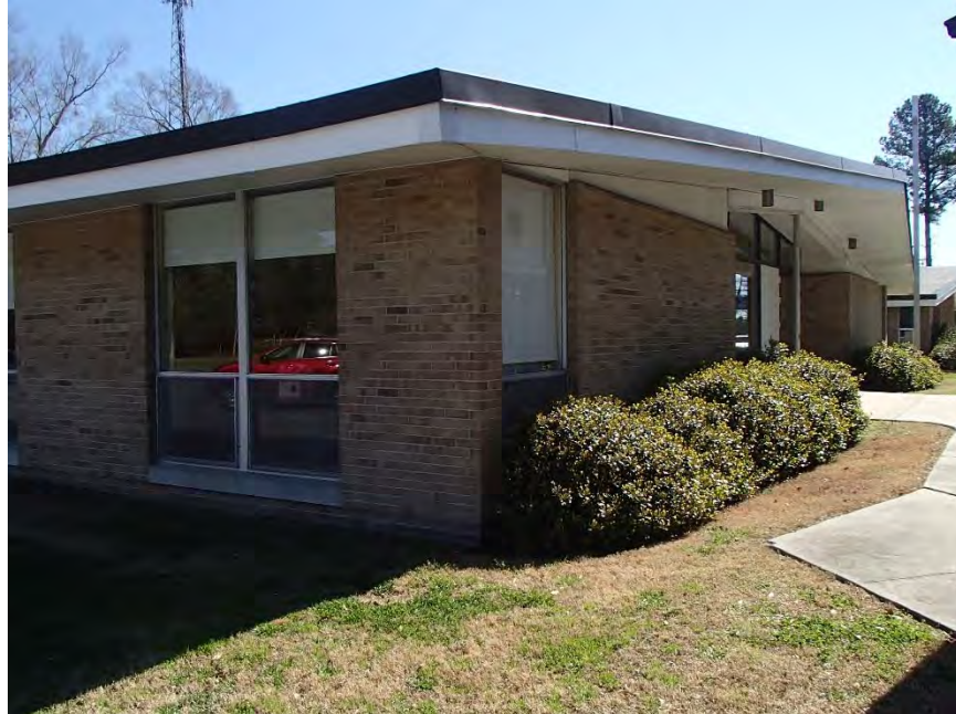
Figure 7: Northwoods UMC, Education Building, west corner
