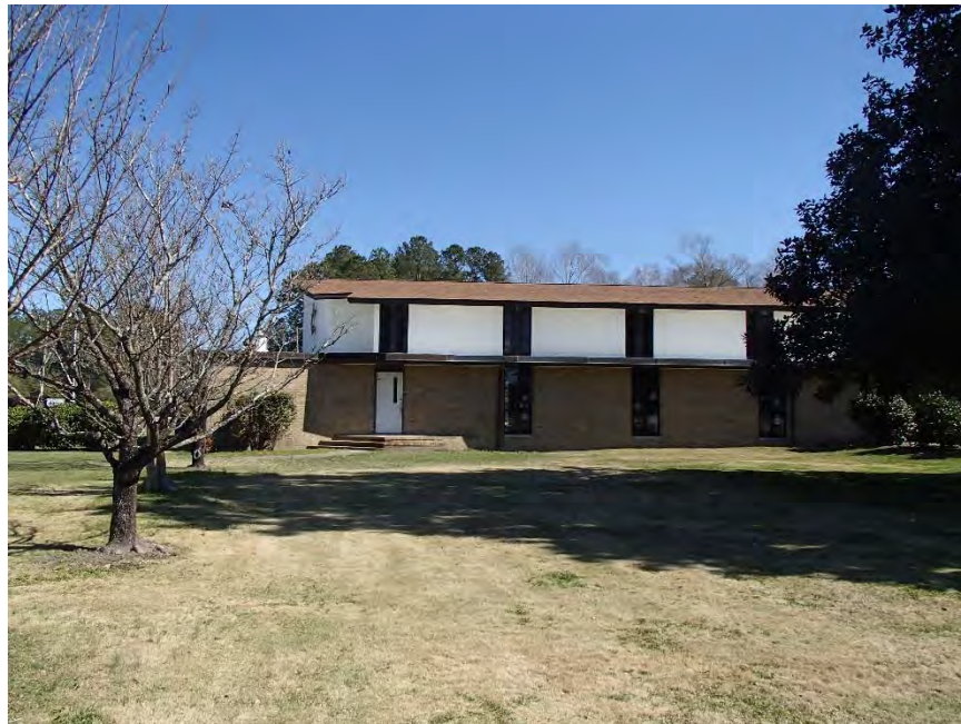
Figure 12: Northwoods UMC, southwest elevation
