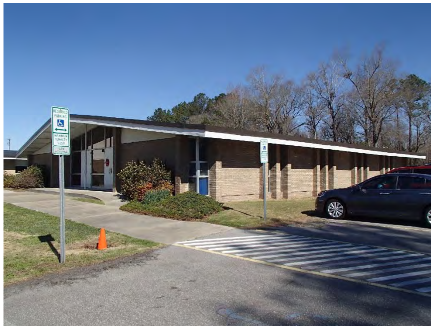
Figure 28: Northwoods UMC, Second Education Building, south corner
