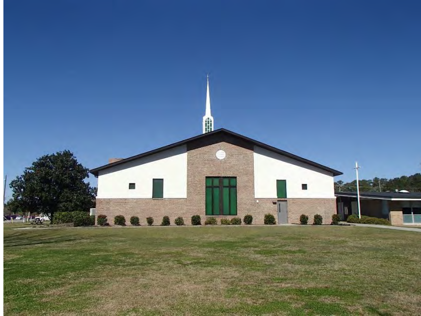
Figure 17: Northwoods UMC, southeast elevation
