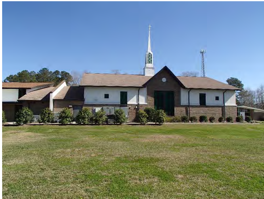
Figure 14: Northwoods UMC, southwest elevation, 2008 sanctuary
