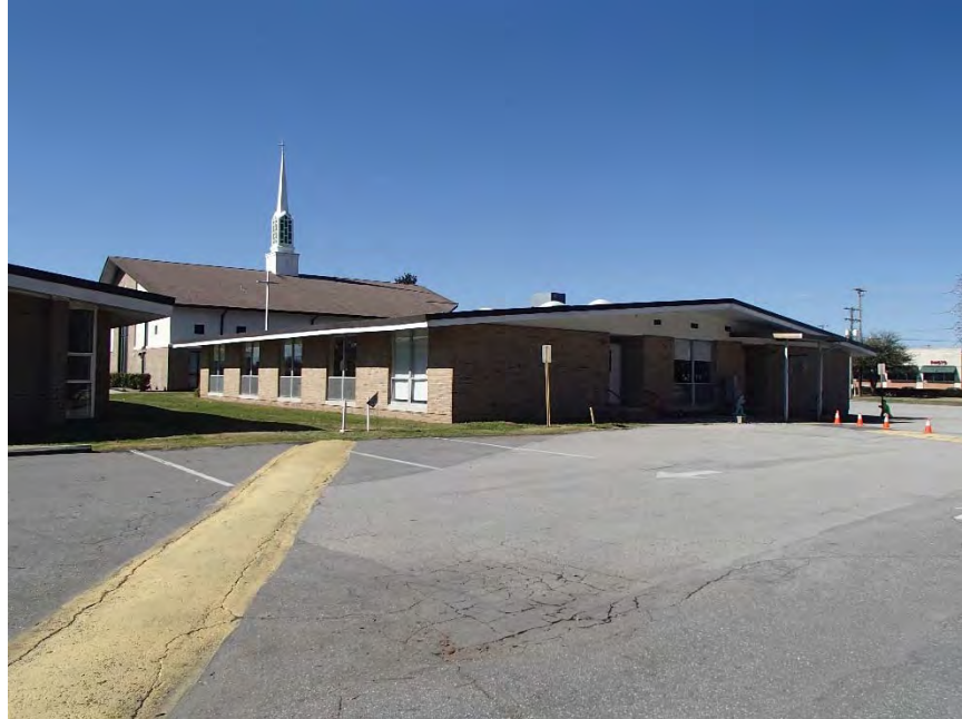
Figure 9: Northwoods UMC, Education Building, northeast elevation
